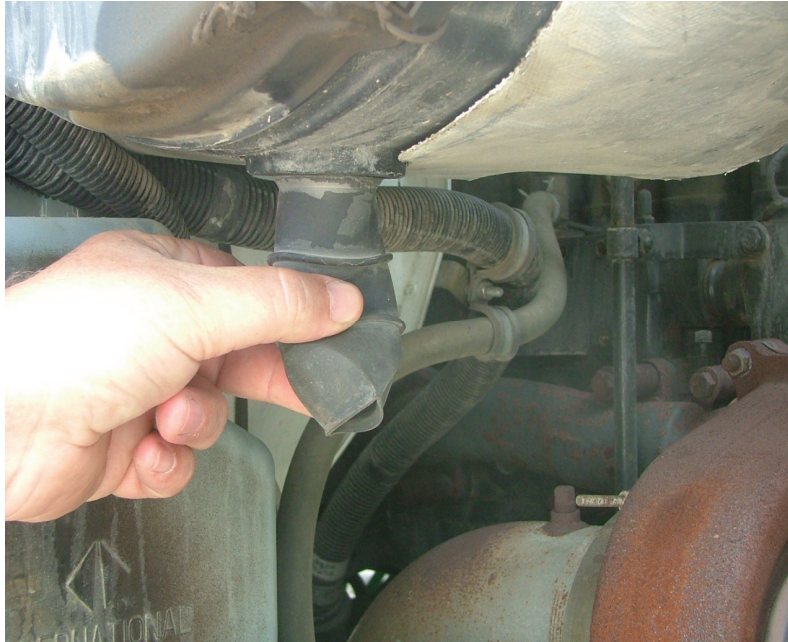
Figure 4-1 Dump truck engine compartment, dirt evacuator
