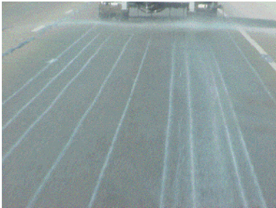
Figure 12-4 Brine being applied
